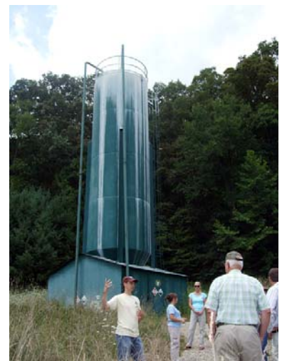
Ben McCament explains how a doser hopper works. (Photo by Larry Porter)
